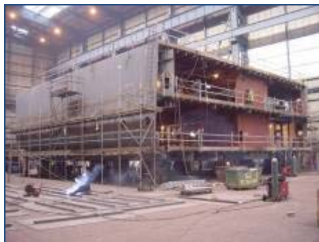
Accommodation unit being fabricated
