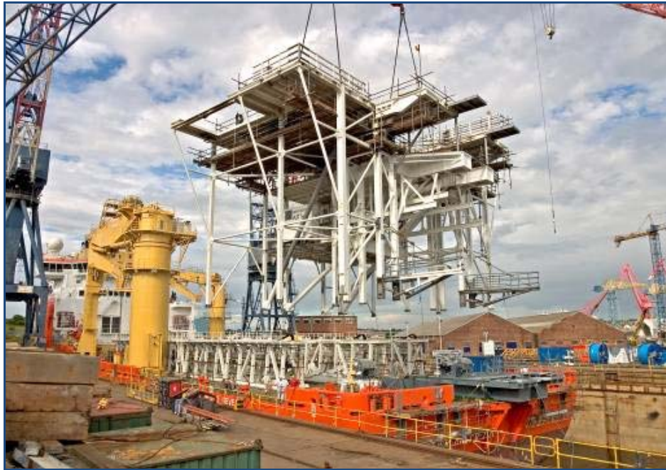
Pre-outfitted module being lifted into position
